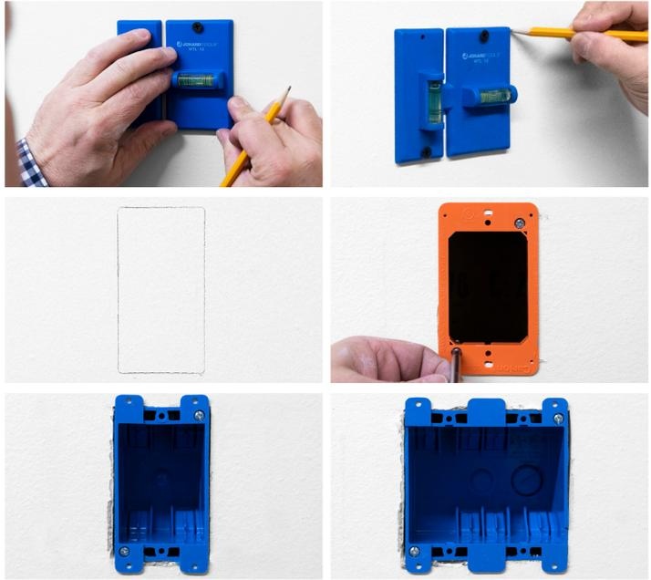
The Jonard Tools WTL-12 is a wallbox template specifically designed for cutting out single and double gang boxes. The built-in levels assist in positioning the template so boxes are straight every time.
